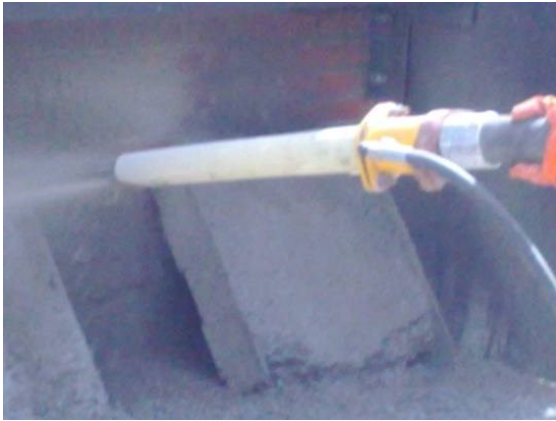
Figure 5. – The working state of the nozzle
