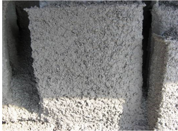
Figure 6. – The large plate after spraying
