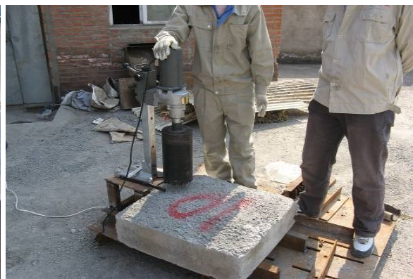
Figure 8. – Slab core drilling
